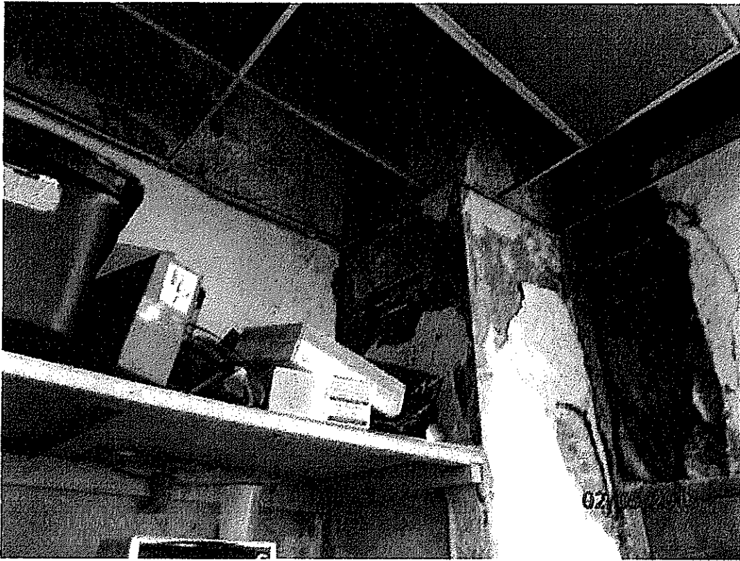
Photo No. 9. Interior Detail 2140 Market Street, Philadelphia, PA
