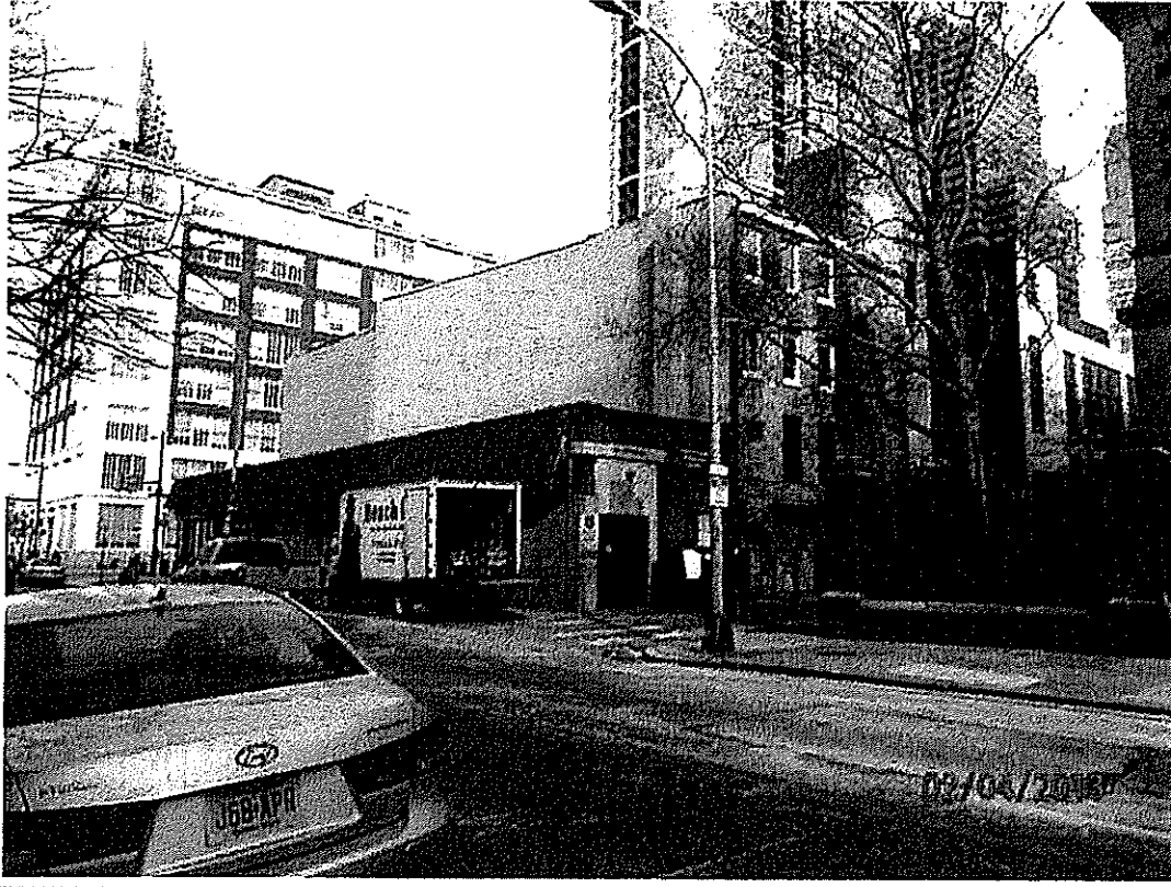
Photo No. 2. Rear (South) View of 2140 Market Street, Philadelphia, PA
