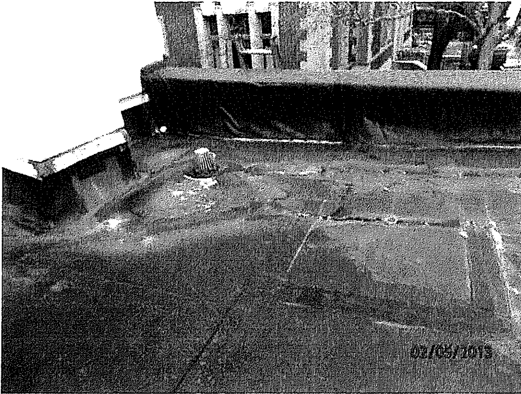
Photo No. 17. Roof View 2140Market Street, Philadelphia, PA
