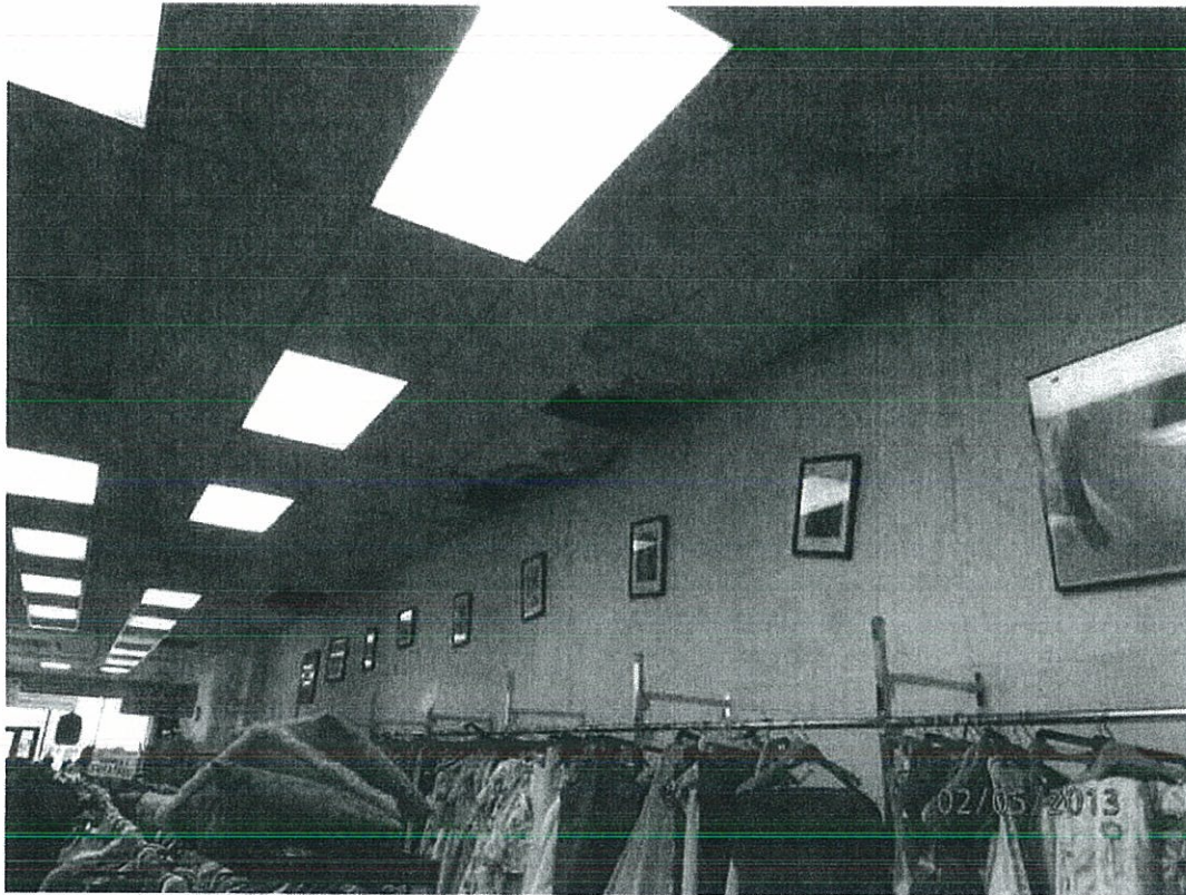
Photo No. 10. Interior Detail 2140 Market Street, Philadelphia, PA
