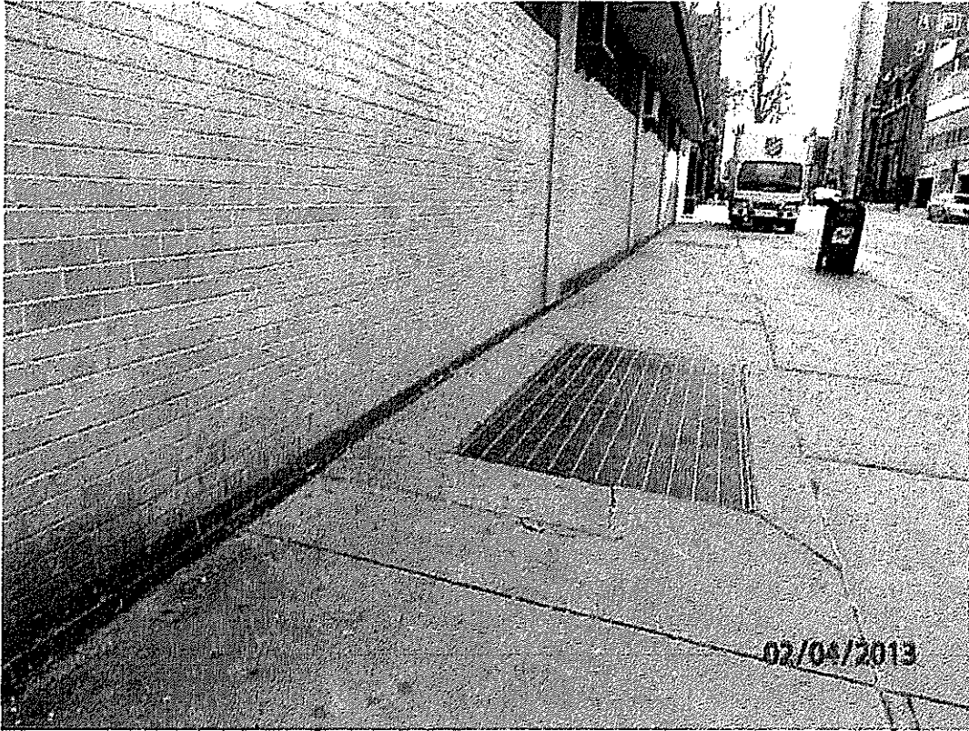
Photo No. 8. Façade Detail 2140 Market Street, Philadelphia, PA
