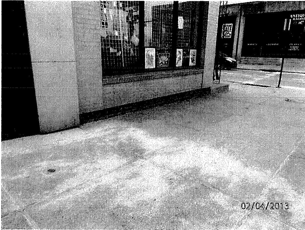
Photo No. 6. Façade Detail 2140 Market Street, Philadelphia, PA
