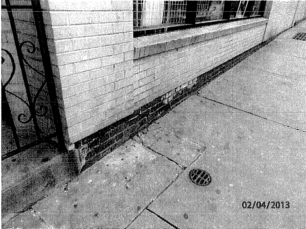
Photo No. 7. Façade Detail 2140 Market Street, Philadelphia, PA
