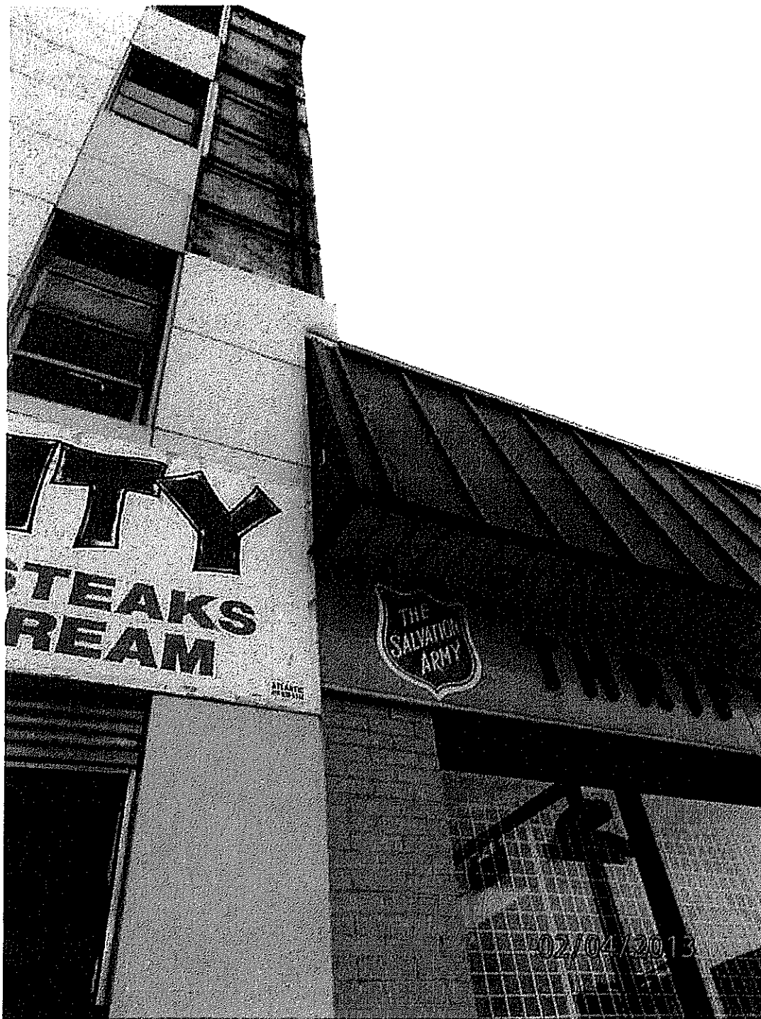
Photo No. 5. Façade Detail 2140 Market Street, Philadelphia, PA
